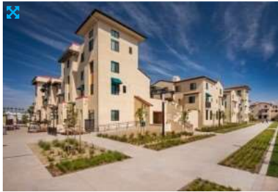
Paradise Creek is home to residents earning between 30% and 50% of the area median income in National City, Calif. Developed by Related California and Community HousingWorks, the new 92-unit second phase joins 109 units completed in the first phase.
