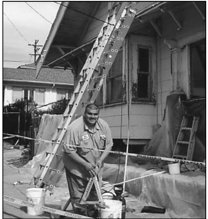
Ramon Hernandez from the Metropolitan Area Advisory Committee (MAAC Project) preps for lead hazard control work on a Sherman Heights home.
