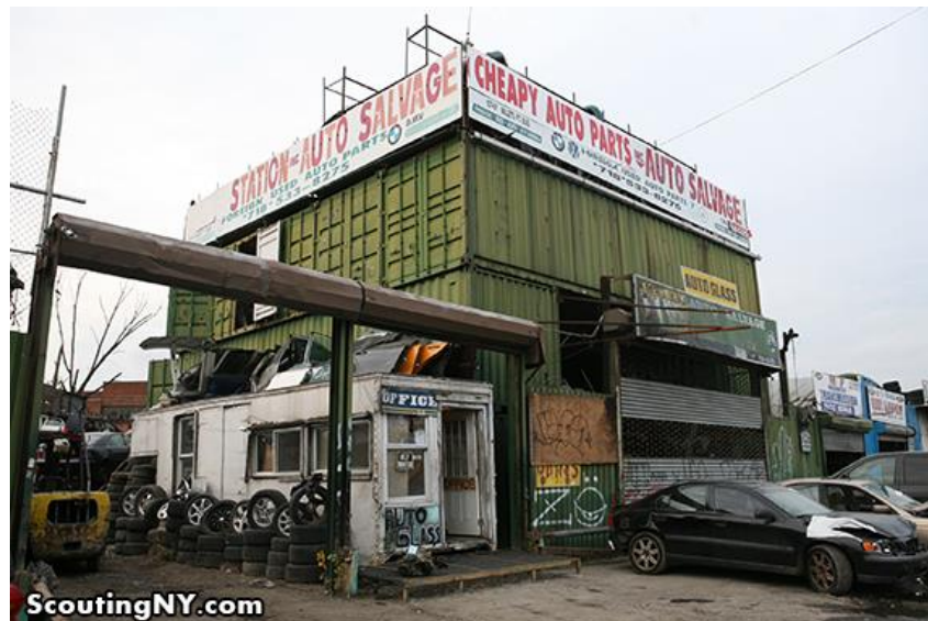
Exterior of Shop Made of Shipping Container
